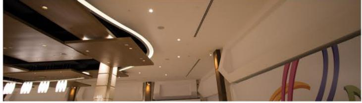
Sonacoustic® acoustical plaster installs seamlessly with other trades and finishes. Costly and obtrusive fixed scaffolding not required, Sonacoustic® is typically installed from a rolling scaffolding, scissor or boom lifts.
